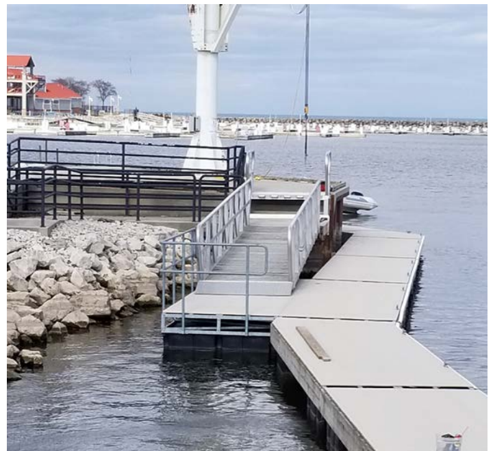
Piers going in. March 18th and 19th.
